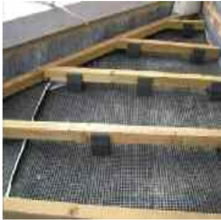
38mm joist shoe with levellers
